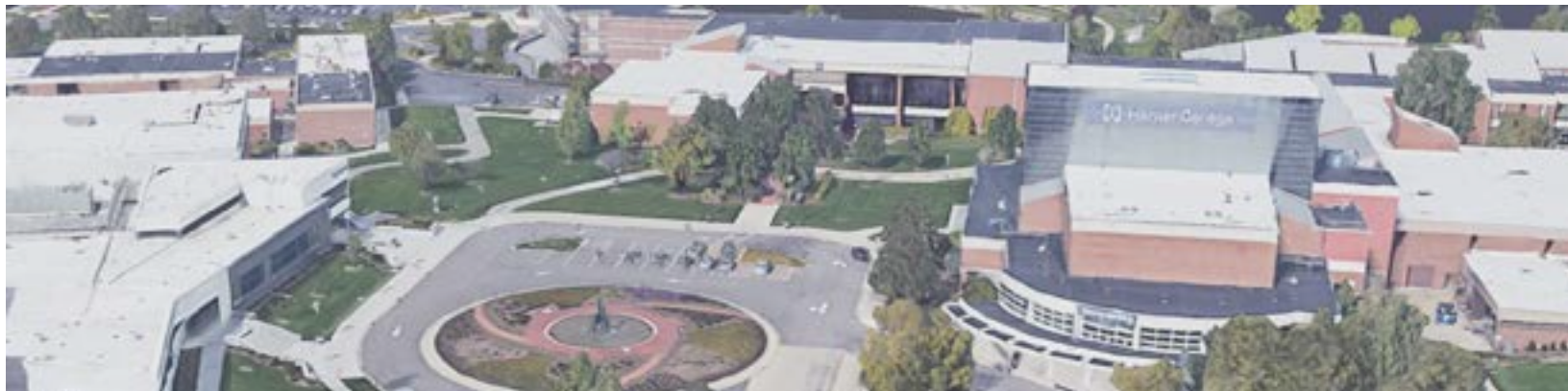
PREVIOUS CONSTRUCTION OUTSIDE BUILDING D
