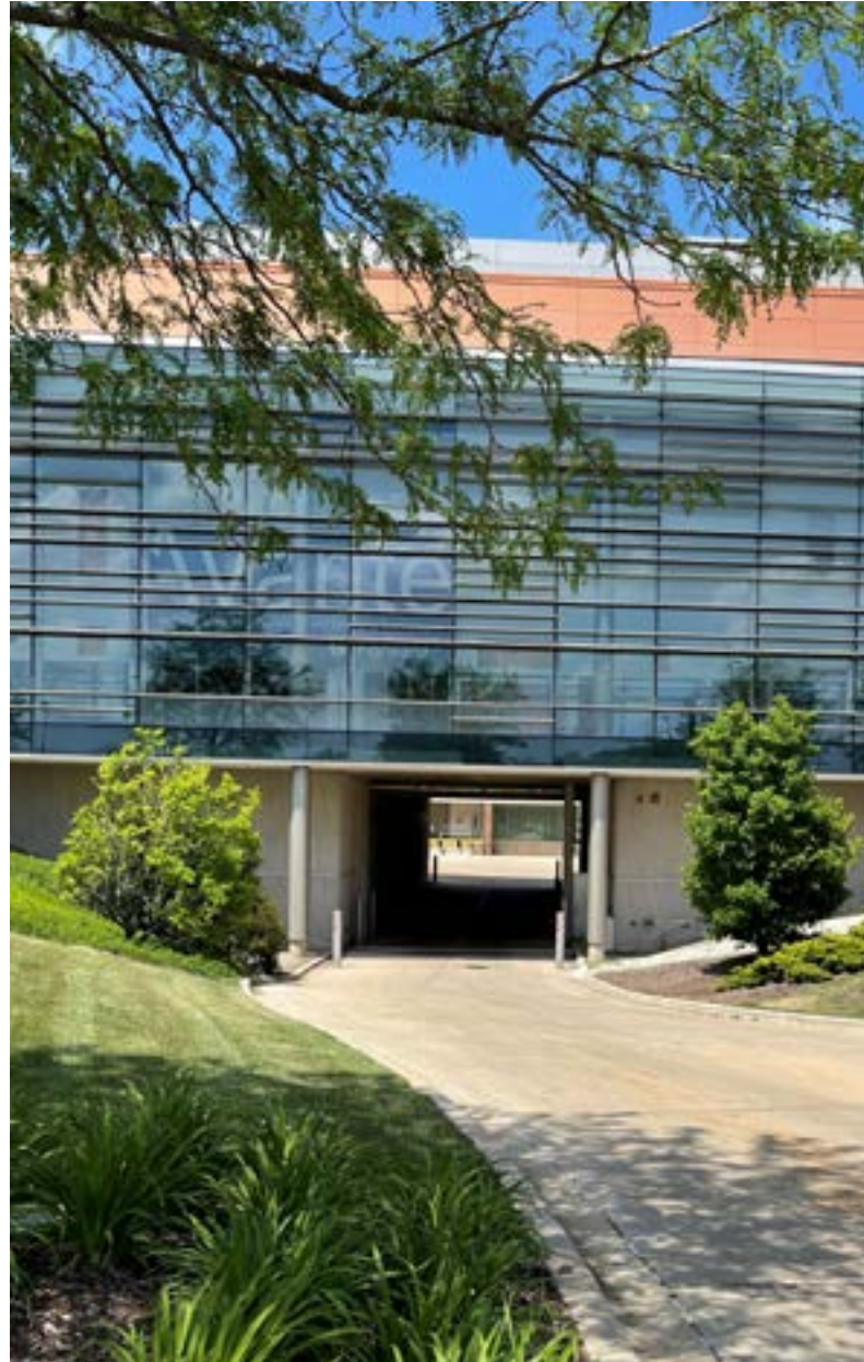
EXISTING SERVICE ENTRY UNDER AVANTE BUILDING
