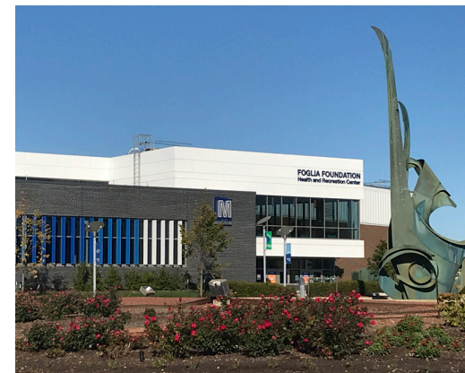
BUILDING M RENOVATION + EXPANSION (2019)
