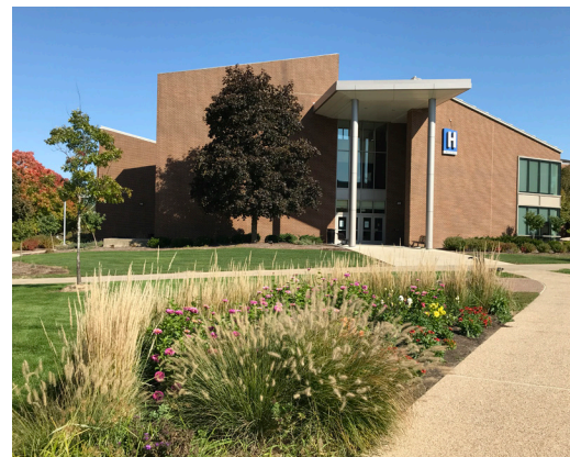
BUILDING H (1977) RENOVATION/ADDITION (2012)
