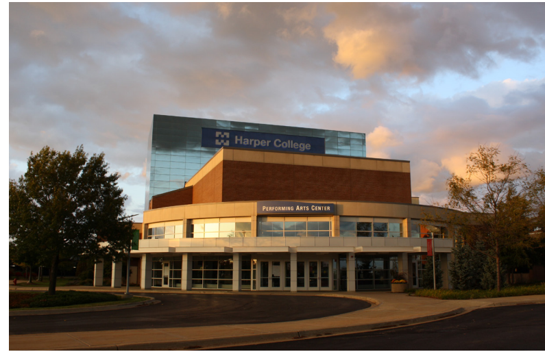
BUILDING R EXTERIOR
