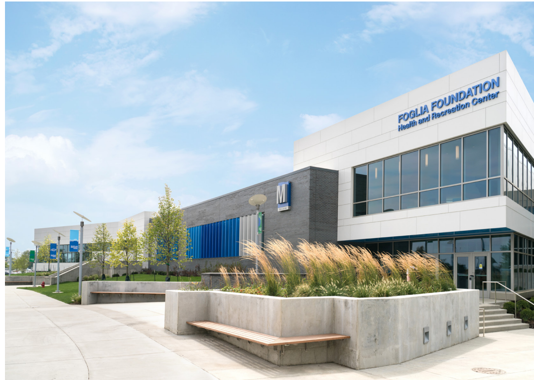
IMPROVEMENTS OF BUILDING M - 2018
