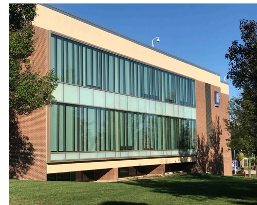
BUILDING F RENOVATION (2018)
