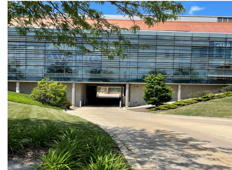
UNDERPASS OF AVANTE TO SERVICE ENTRY
