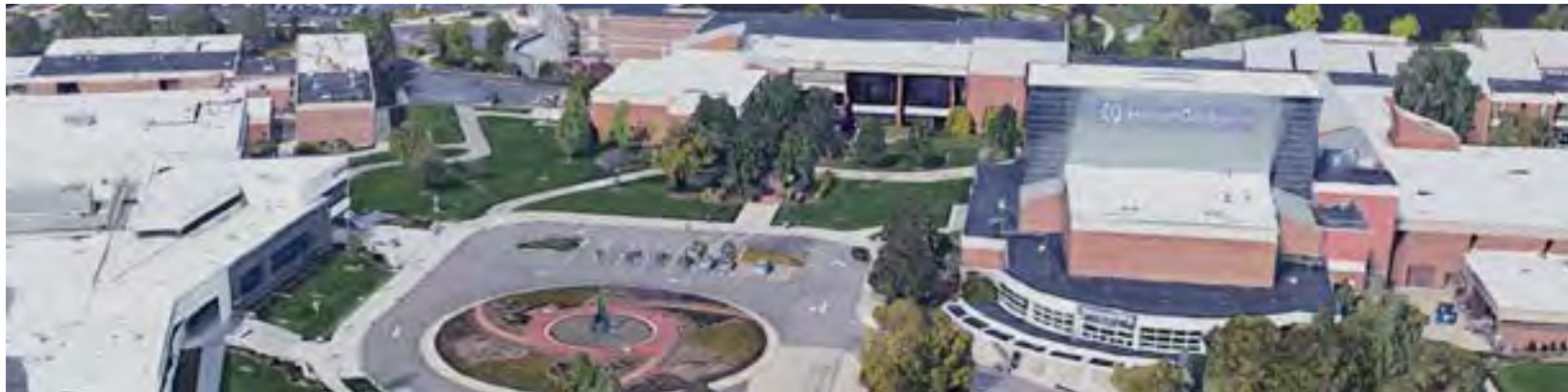
PREVIOUS CONSTRUCTION OUTSIDE BUILDING D
